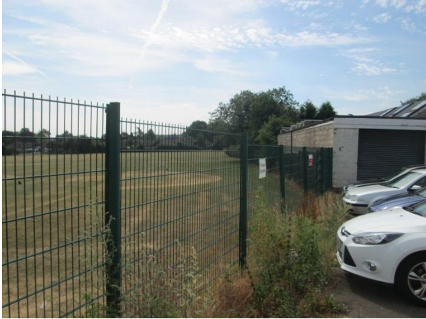
Rear boundary with adjacent Kimberley School
